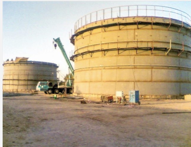
Construction of Condensate Storage Tanks API 650; self-supported cone roof with pontoon type internal floating roof and associated piping at Bubak Sehwan Gas Field, Sindh, Pakistan.
