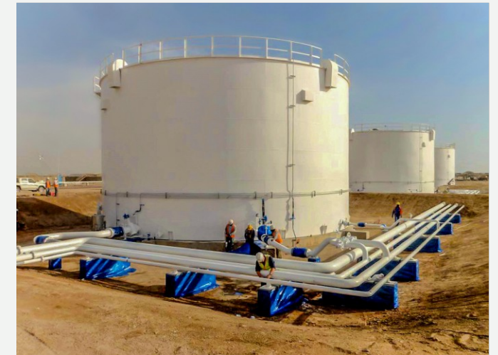
Engineering, Procurement and Construction of three (03) API-650/620 JP-8 Fuel, self-supported, honeycomb type floating roof storage tanks in Helmand Province, Afghanistan.
