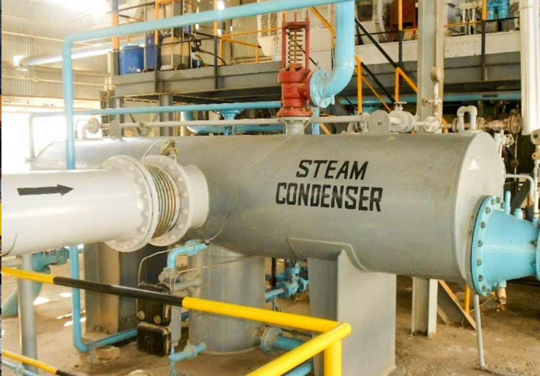
Manufacturing of Vacuum Condensers of Turbo Generator No.7 Installed at Sui Purification Plant; Type: Straight Tube, Pressure: 6 bar / -17.2 bar (tube / shell) Tube Size: 14mm (Qty. 644), Material: CuNi10Fe1Mn F29
