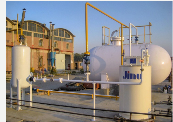
Supply of SNG systems comprising of 3.5ton LPG Tanks, Air & SNG Tanks and Vaporizers at Shahkam Industries (Pvt.) Ltd., Pakistan.
