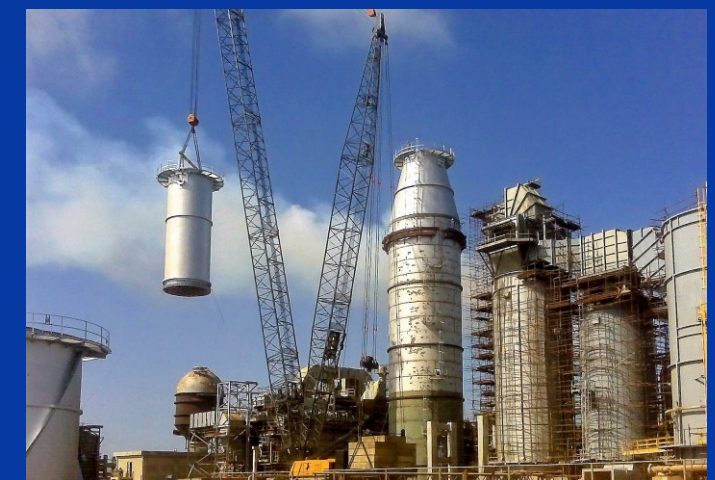
Erection of 97 meter / 410 ton stack at BYCO Refinery, Pakistan.
