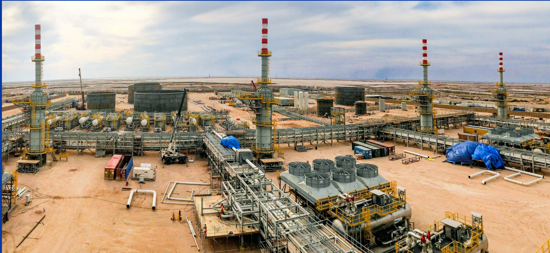
Construction of twenty-one (21) API-650 Crude oil, self-supported, dome roof storage tanks, at Initial Production Facilities (IPF) Hammar, Zubair and Rafidiyah at Zubair Oilfield in Iraq.
