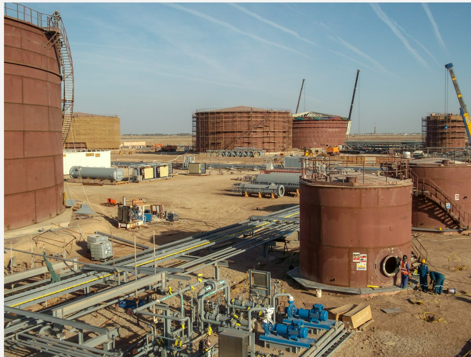
Construction of eight (08) API-650 Crude oil, self-supported, cone roof storage tanks, plant piping, structure and plant erection at First Commercial Production Facility at Garraf Oilfield in Iraq.
