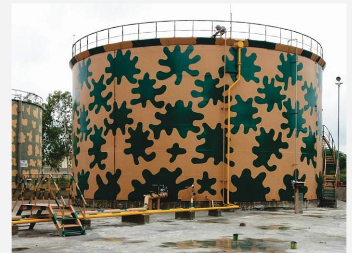
Engineering, Procurement and Construction of API-650 storage tank at Pakistan Petroleum Limited's Adhi Gas Field in Pakistan.
